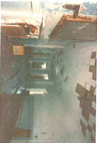
Trinity House, Before Renovations
